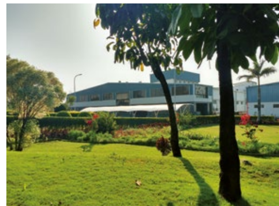
Exterior view of the plant
